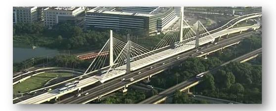
**Description:** The Ayrton Senna Stayed Bridge is 200 m long and located in Barra da Tijuca borough of Rio de Janeiro. The foundations consisted of 2 m diameter bored piles excavated through soft clays and sands to the top of the bedrock. Then, they were pinned to the rock using root piles.
