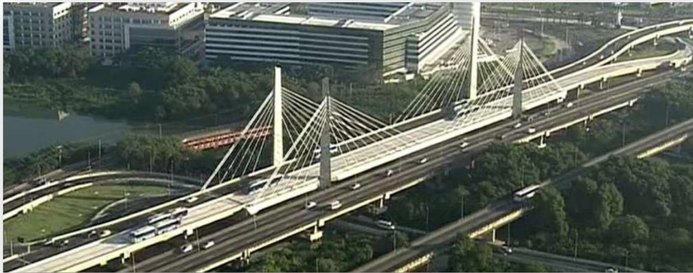
**Description:** The Ayton Senna Stayed Bridge is 200 m long and located in Barra da Tijuca borough of Rio de Janeiro. The foundations consisted of 2 m diameter bored piles excavated through soft clays and sands to the top of the bedrock. Then, they were pinned to the rock using root piles.
