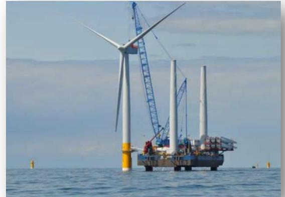
**Description:** The scope of the work was the spectral analysis of dynamic monitoring carried out by the client of one offshore wind turbine. Terratek processed the data using advanced dynamic techniques, such as SSI *stochastic subspace identification*, yielding spectrum and damping values. Terratek studies also yielded horizontal displacements at the top of the monopile level which was below 1 mm, much less than the maximum expected and below the level that may yield to cyclic mobility.
